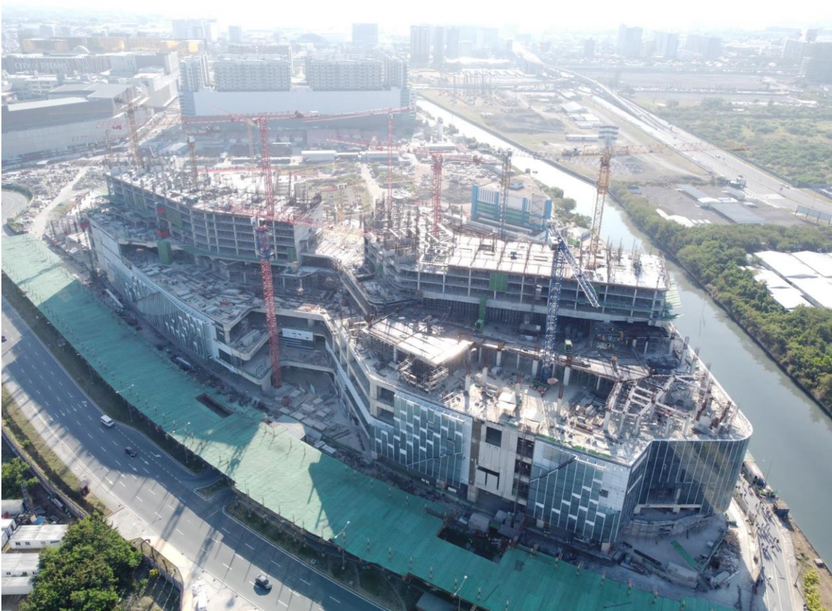
Figure 1 Construction progress at Westside City Project in March 2023
